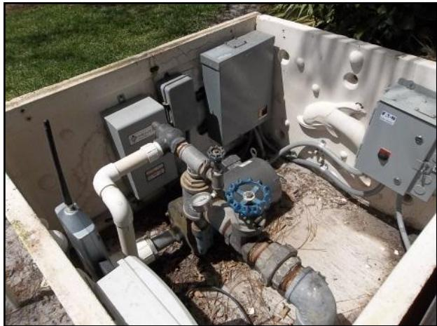
**Figure 7: Pump housing walls are not sturdy.**
