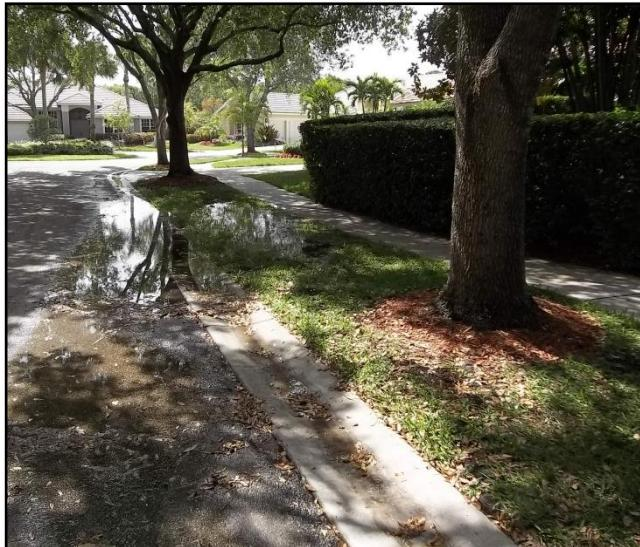
**Figure 5: Tree roots causing improper drainage.**
