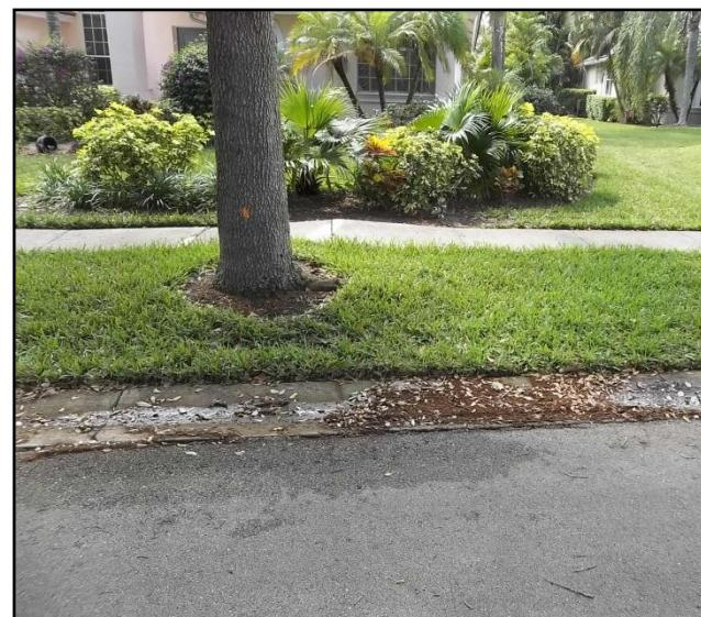
**Figure 4: Tree roots causing sidewalk to heave.**
