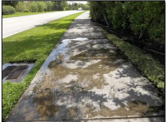
**Figure 6: Water standing on sidewalk from a possible irrigation leak.**
