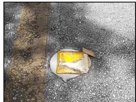
**Figures 2 and 2:** Storage shed needs painting and pavement reflectors need replacement.
